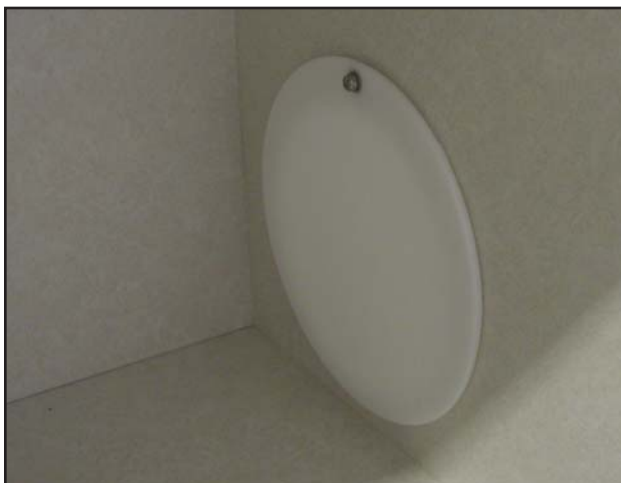
Figure 20B. Completed Kitty Suite Port Hole Installation
