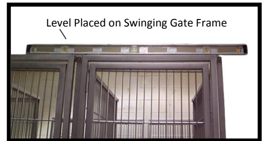
Figure 36: Checking left-to-right level
