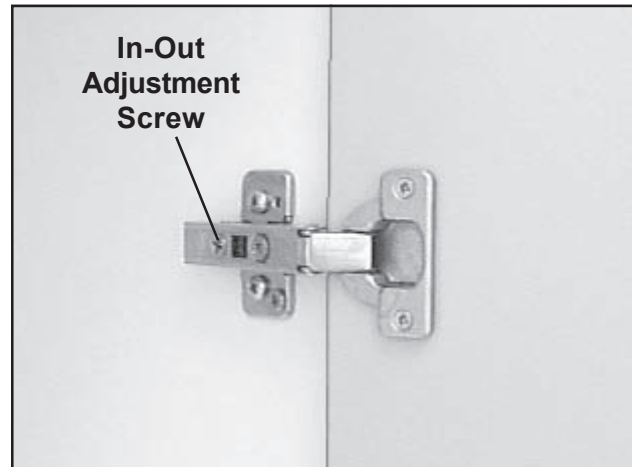
Figure 13. Door In-Out Adjustment Screw
