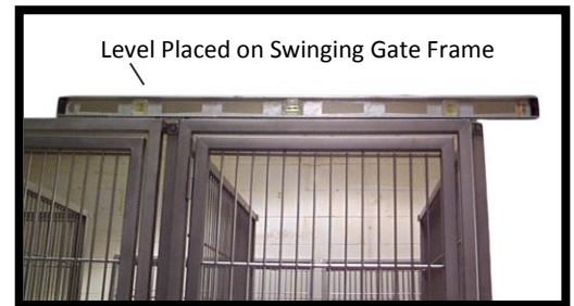
Figure 33: Checking left-to-right level
