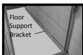
Figure 29: Floor Support Bracket on Facility Wall
